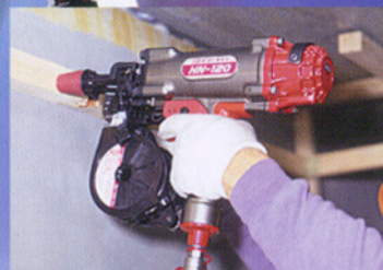
Wood Track to Concrete Wall
